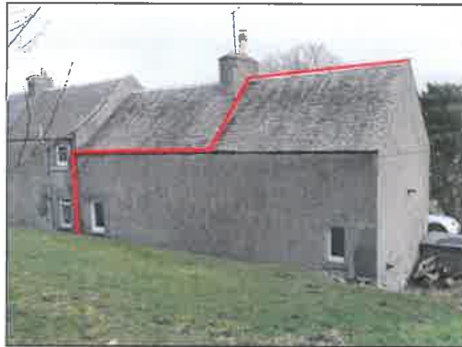
Fig 3: North elevation of the cottage (extent of accommodation outlined in red)
