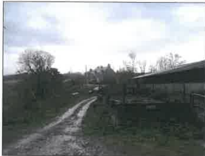
Fig. 12: Agricultural access leading to rear (east) of farm buildings
