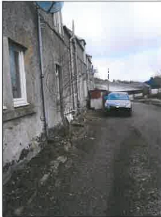
Fig 4: External circulation space
