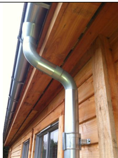
Fig 2 Proposed timber cladding + rainwater goods
