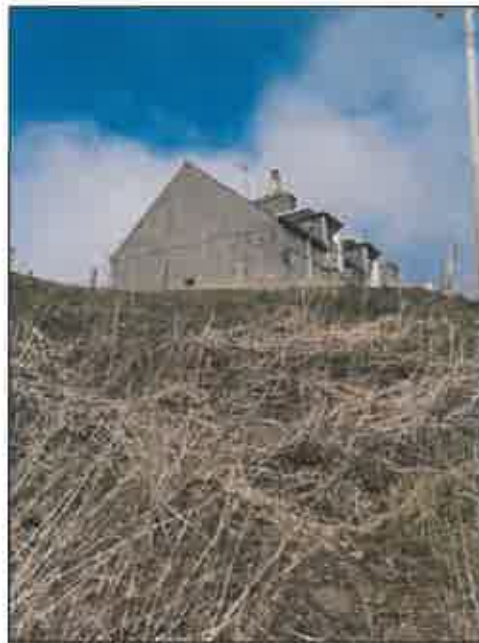
Fig 8: Steep land immediately to the south
