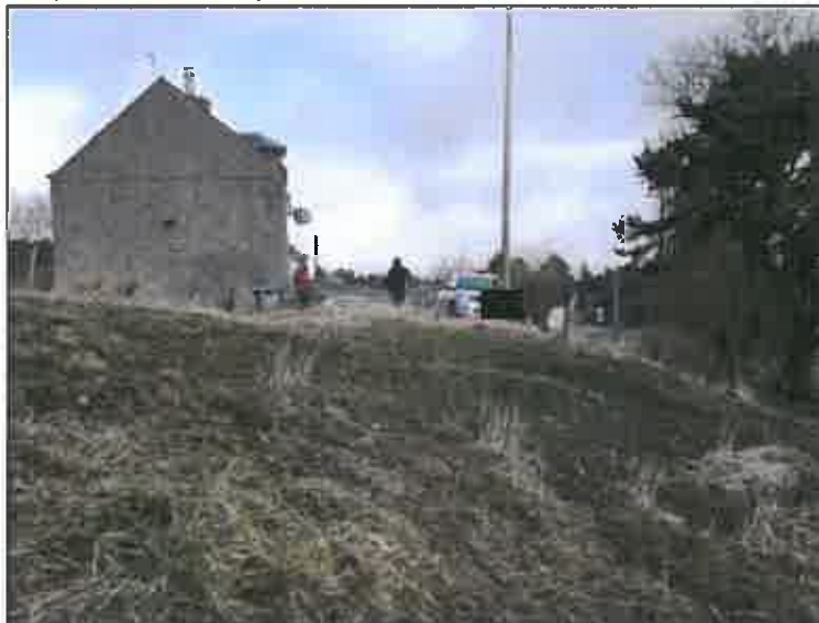
Fig 6: Steep land immediately to the south
