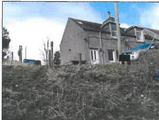
Fig 7: View of southern elevation
