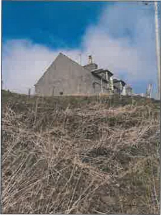
Fig 7: Steep land immediately to the south
